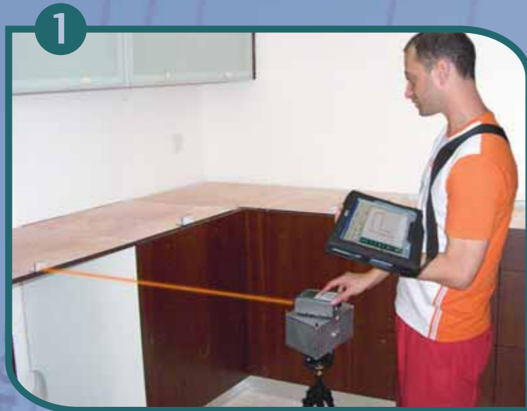
1 The measure person draws and takes measurements in an easy point-and-click process using the InnoDraw laser system.
